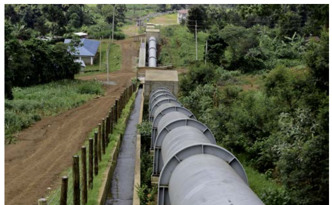
Metumi small hydropower plant canal
