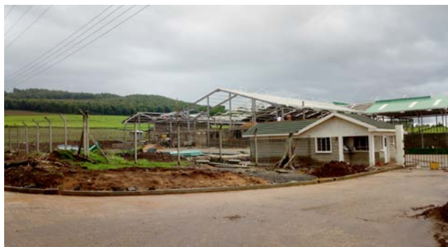
Ongoing construction of Kangaita research factory
