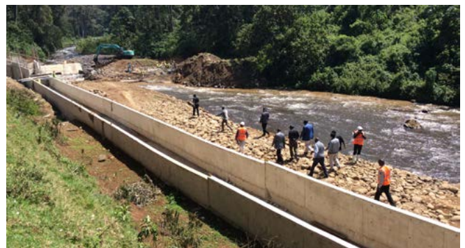
Complete canal at Gura SHP
