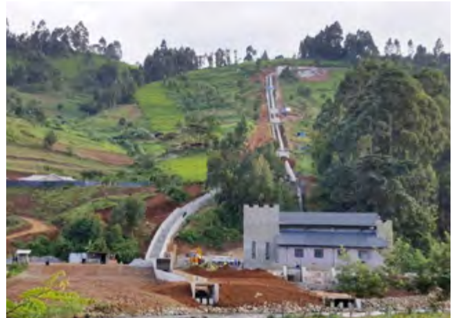
Gura Hydro – Penstock & Power House
