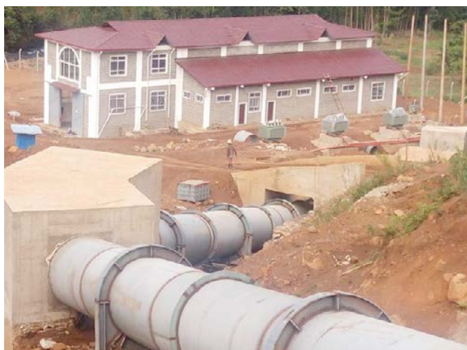
Ongoing construction of North Mathioya hydropower
