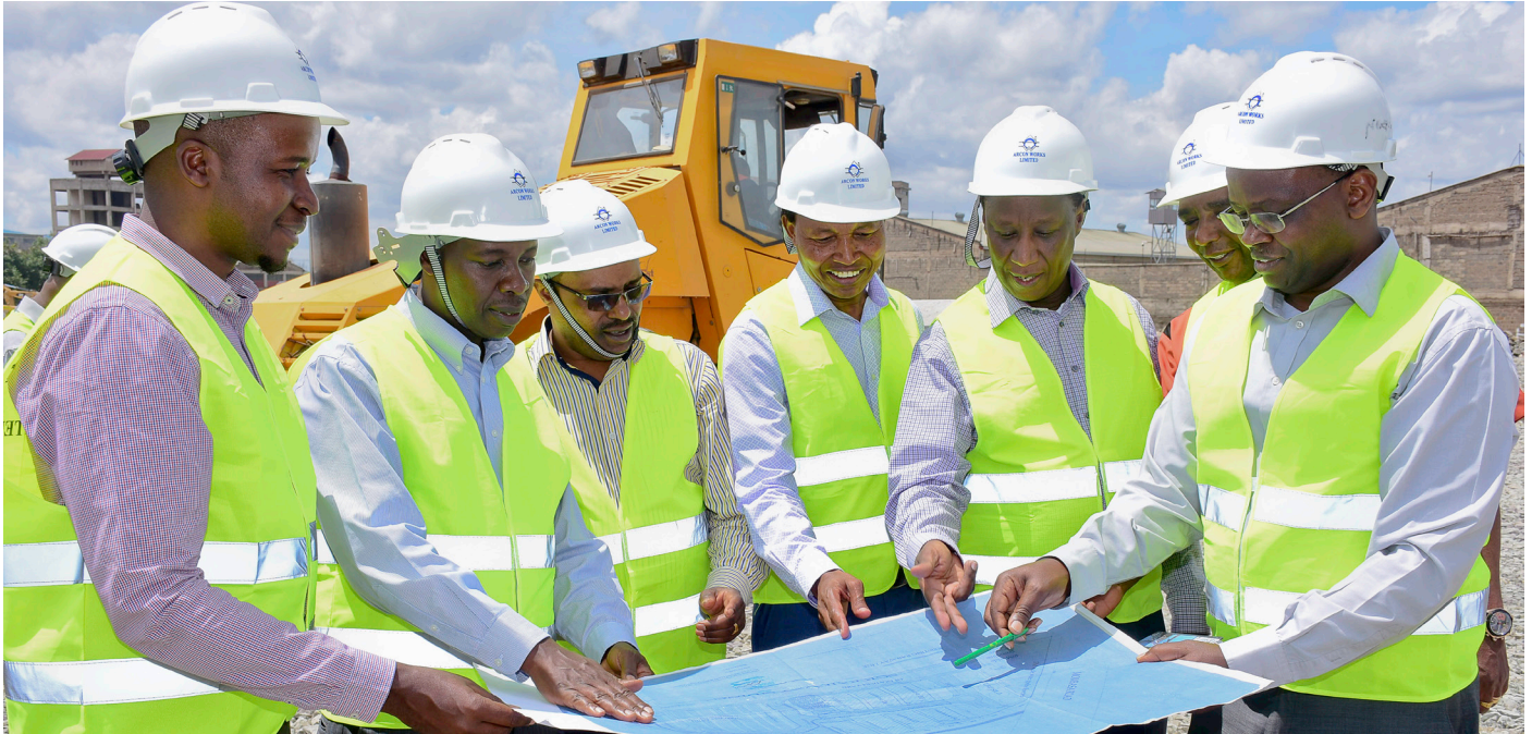
Senior KTDA management, led by Group CEO, Lerionka Tiampati, and Arcon Works Limited Managing Director Joseph Maina (4th From Right), inspect the architectural plans for the proposed Chai Logistics Centre that is being constructed adjacent to the Inland Container Depot - Nairobi, along Mombasa road.
